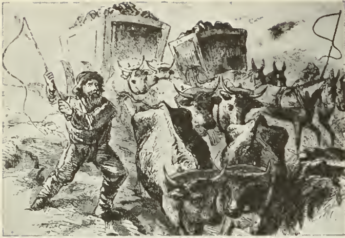
HAULING ORE FROM THE MINES—The difficulty of transporting ore from mines to furnaces and lead from furnaces to markets, over miserable roads and across unbridged streams, accentuated the need for railroads. From Harper's New Monthly Magazine , June, 1865, by courtesy of Harper's Magazine .
