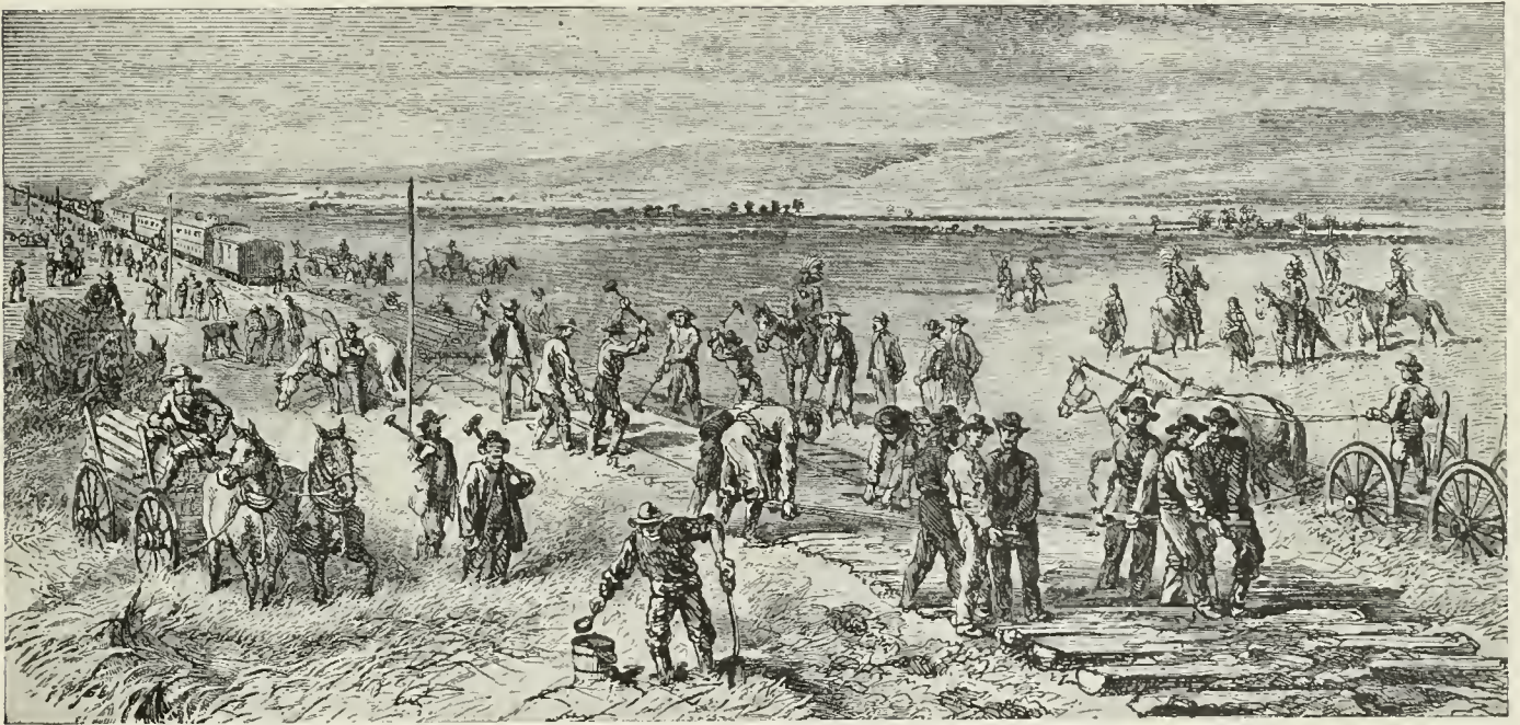
TYPICAL RAILWAY CONSTRUCTION SCENE—The building of a railroad across the sparsely settled prairies was a formidable undertaking in the early days. There were then no powerful steam shovels or track-laying machines to perform the prodigious tasks.
