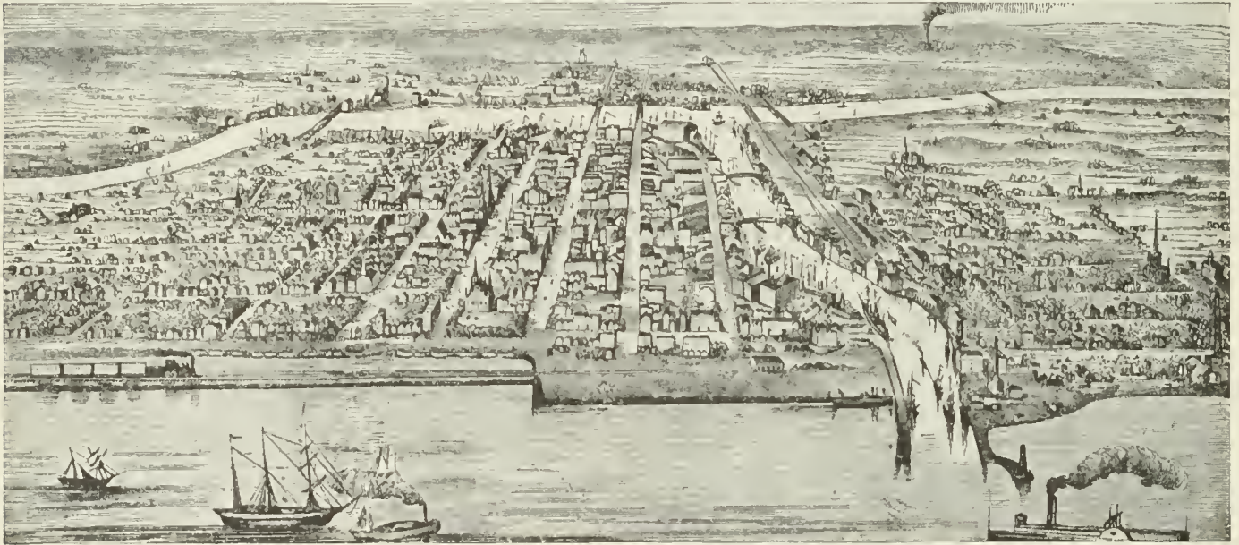
CHICAGO IN 1853—The Illinois Central originally entered the city on a trestle in the lake. This location was designated by the city council in order to relieve the city of the heavy expense of protecting the shore line against lake storms. The railroad built a breakwater at a cost to itself, and a saving to the city, of millions of dollars.
